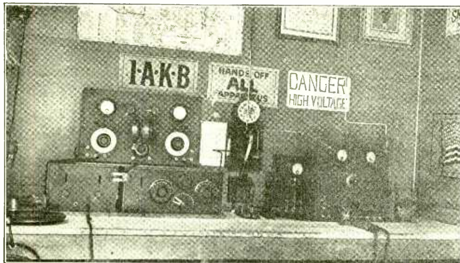
1AKB Is One of the Stations That Was Heard in France During the Trans-Atlantic Tests. The Absence of Helter-Skelter Wiring Is a Point to the Credit of Mr. Cucuvalas, the Owner. Note That the Wiring of the Receiving Units Is From Right to Left. This Allows Short Leads to the Antenna Switch.
