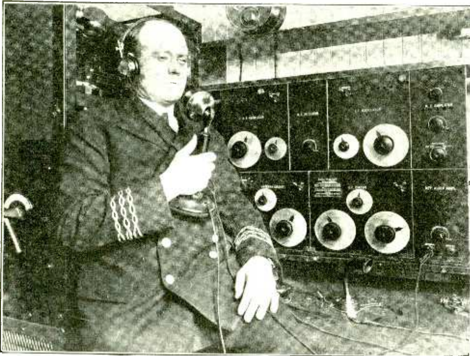
A Splendid View of the Receiving Apparatus Aboard the S.S. Leviathan. To the Left Is an Eight-Tube Duplex High-Speed Receiver, and to the Right an Eight-Tube Navy Standard Long-Wave Receiver.
